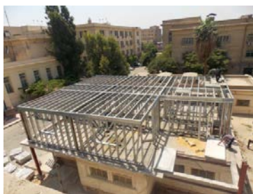
CFS Digital Library Building at Cairo University during Construction
