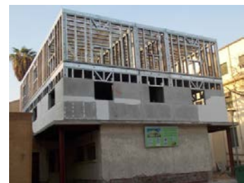
CFS Digital Library Building at Cairo University during Construction
