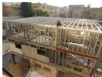
CFS Digital Library Building at Cairo University during Construction
